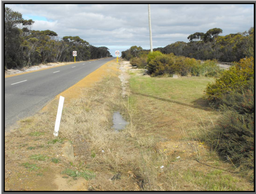
Image 6: Open and unsightly drains on South Coast Highway
